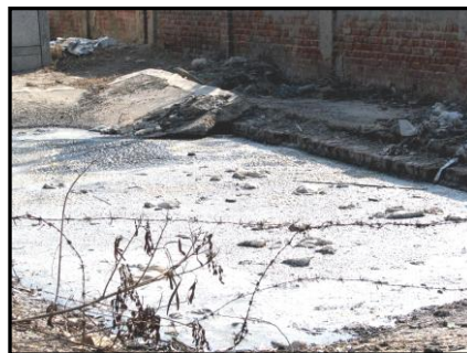
A collapsed toilet block leaves the slum with an open septic tank
